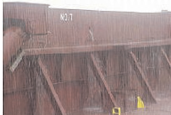
Hose testing and a typical hose test
