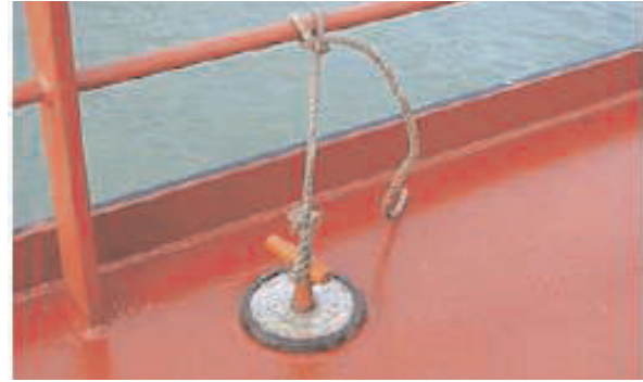
Scupper plug fitted
