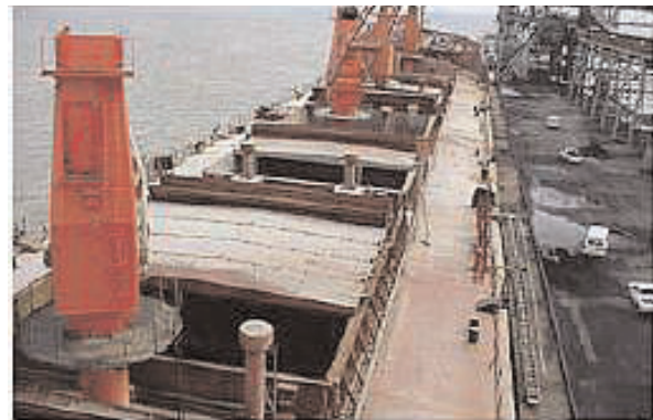
Cement staining on decks and hatchcovers
