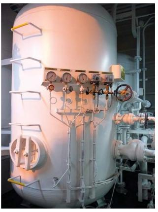
Depleted air bottles: Excessive numbers of engine starts/ stops during manoeuvring will deplete pressure in the main engine start bottles which can result in loss of control of the vessel at critical times, such as when docking, due to the engine failing to start.
