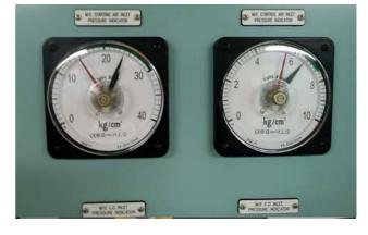
Good start air pressure with safe operational limits marked
