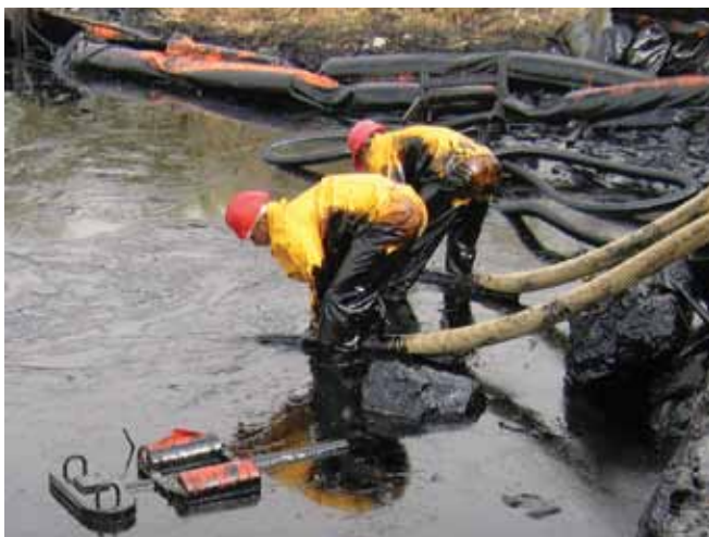
▲ Figure 10: Workers placing a hose attached to a vacuum pump directly into the oil. In this instance, the small weir attachment has been removed to allow the viscous fuel oil to flow into the hose, with a consequent potential increase in entrained water.
