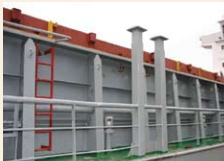
Permanent ladder with backfall protection
