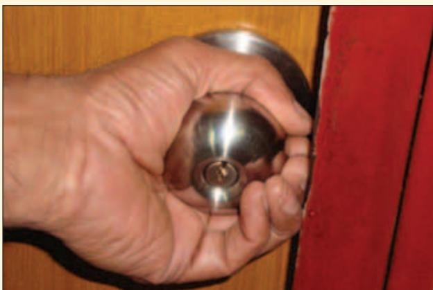
▲ Figure 4: Doorknob fitted too close to doorway frame, risking crush injuries to fingers. Lever-activated door latches will keep fingers away from the door edge.
