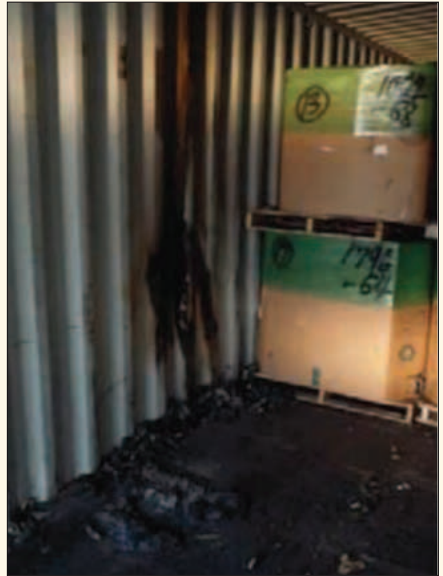
▲ Figure 6: Heat damage to inner surface of container's side panel
