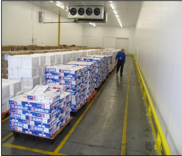
Cargo should be held at the required temperature and correctly stowed in the cold rooms in order to facilitate adequate air flow management and optimal temperature management while being stored at the receiving warehouse.
