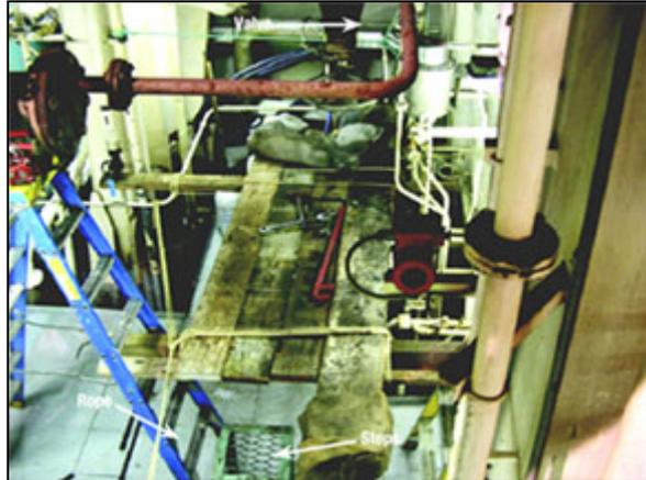
In an effort to escape the hot water spray the chief engineer tried to jump clear of the staging but became entangled in the ropes securing the staging; he had one leg either side of the securing rope and had fallen forward. The report concludes that
