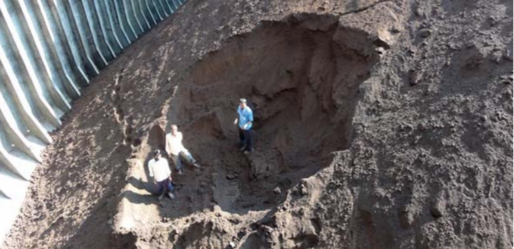
it may be sufficient to manually excavate sampling pits to a depth of about 50cm. Where the stow is deeper, it is preferable to utilise the ship's gear with a grab to excavate deeper pits and to draw samples from these – providing of course that the barge is alongside a geared vessel.
