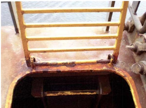
If visual inspection of these features reveals corrosion or wear, effective maintenance should take place at the first opportunity. It should also be noted that the wear to the protective paint coatings should be rectified quickly as these will precipitate the metal corrosion process if left untreated.
