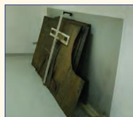
▲ Ineffective securing arrangement of plate storage rack
