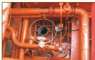
▲ Figure 1: View of open Butterworth hatch
