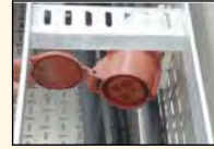
▲ Protected female sockets replaced male plugs for power supply cables
