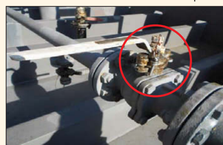
▲ Tank cleaning line supply valve – note missing locking pin
