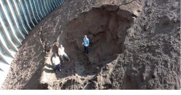
it may be sufficient to manually excavate sampling pits to a depth of about 50cm. Where the stow is deeper, it is preferable to utilise the ship's gear with a grab to excavate deeper pits and to draw samples from these – providing of course that the barge is alongside a geared vessel.
