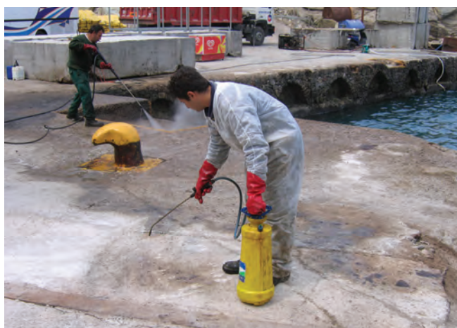
▲ Figure 23: A chemical shoreline cleaner applied to an oil stain followed by pressure washing.
