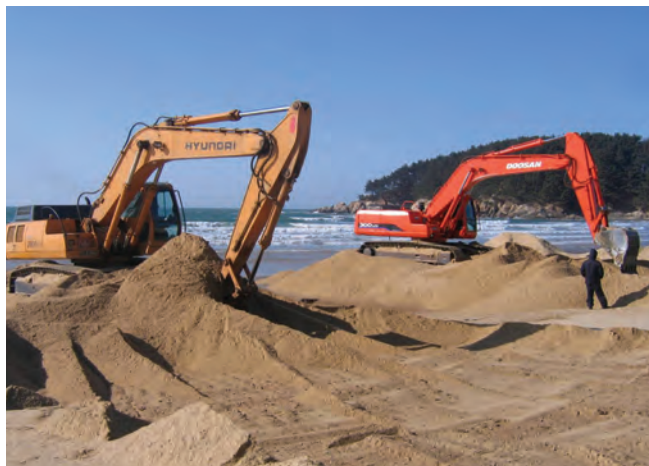
▲ Figure 18: Lightly contaminated sand is moved to the intertidal surf zone for washing on subsequent tides.
