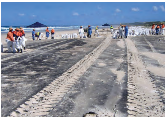
▲ Figure 6: The use of machinery on oiled shorelines can lead to additional contamination. Here, tractors have driven over an area of oil, forcing the oil into the beach.
