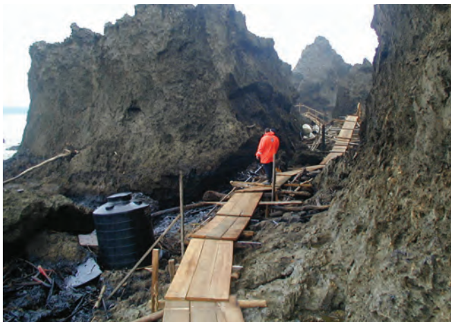
▲ Figure 35: To minimise hazards to workers on rocky shorelines, temporary walkways can be constructed.
