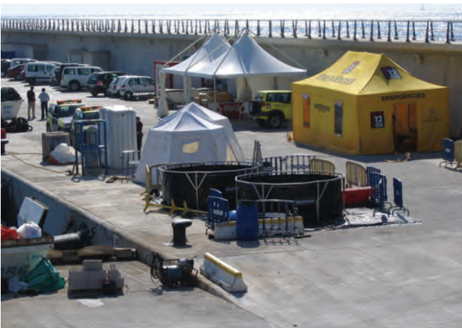
▲ Figure 45: Temporary buildings sited close to a work site provide catering and sanitary facilities for the workers.
