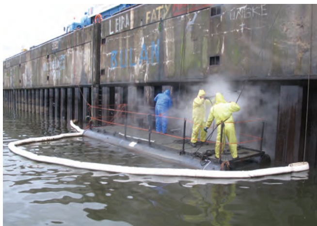
▲ Figure 30: Oiled pilings and dock quay being pressure washed from a small raft. Released oil is collected in the sorbent boom.
