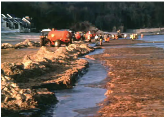
▲ Figure 4: Agricultural vacuum tankers recovering oil that has been pushed and flushed into trenches.
