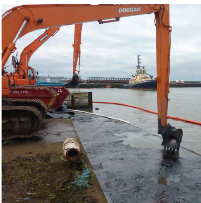
▲ Figure 5: Civil engineering machinery employed to recover oil from a port area. In this situation, the water temperature was below the pour point of the oil, causing the oil to become semi-solid, precluding the use of skimmers.
