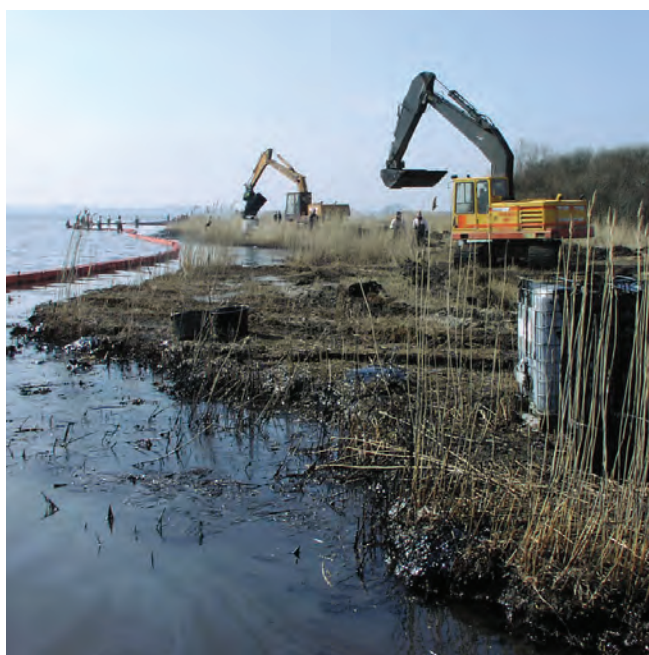
▲ Figure 41: Use of heavy machinery on sensitive areas of the shoreline may cause considerable additional damage. In this case, the need to rapidly recover free-floating oil was a priority.
