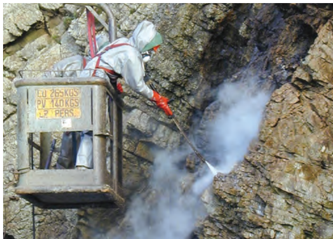
▲ Figure 21: Pressure washing a cliff face above an amenity beach. The oil was thrown high up the cliff in a storm and without cleaning would be likely to persist for some time.
