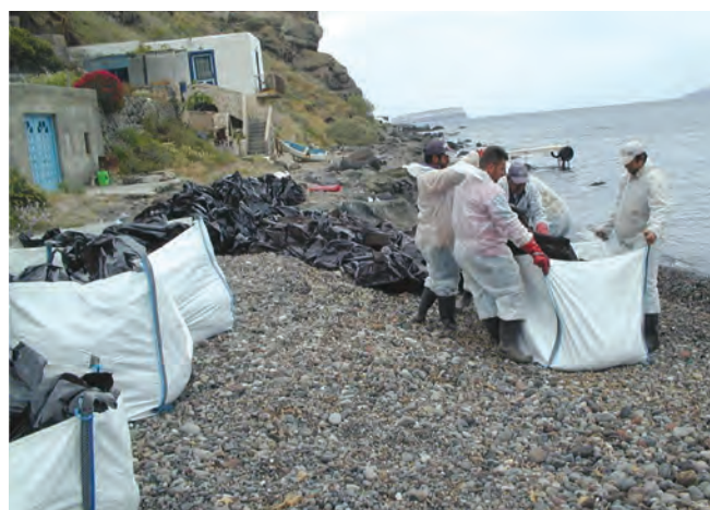
▲ Figure 10: Small bags of waste are consolidated into larger one tonne 'big-bags' for ease of transport to disposal.
