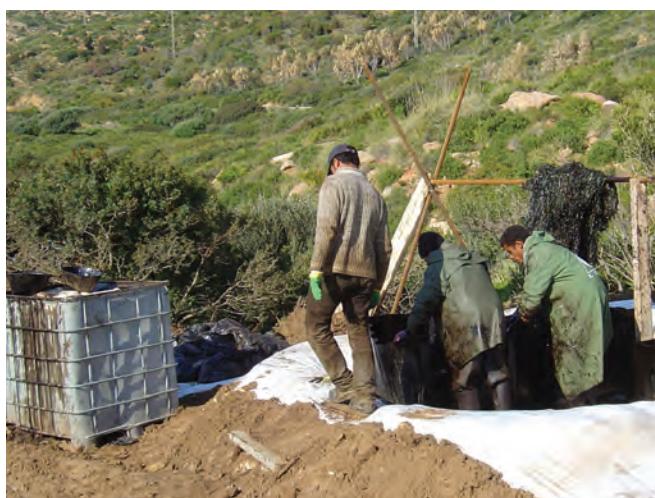
▲ Figure 16: Recovered sorbent snare hung on a pole to allow oil to run into a container, thereby minimising the amount of free oil in the waste.
