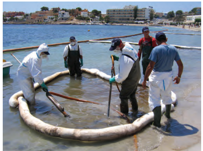
▲ Figure 1: Polypropylene sorbent boom used to collect oil released during flushing operations.
