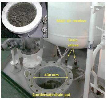
Drainage pot arrangement. Inset shows observation glass in place.
