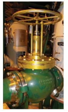
Spindle valve assembly
