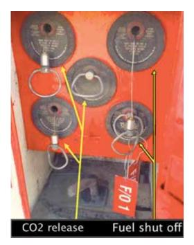
activated what he thought was the fuel oil shut-off but instead the CO2 was released. Fortunately, the audible alarm system and release time delay functioned as intended, allowing personnel to safely evacuate the machinery spaces prior to the CO2 discharge.
