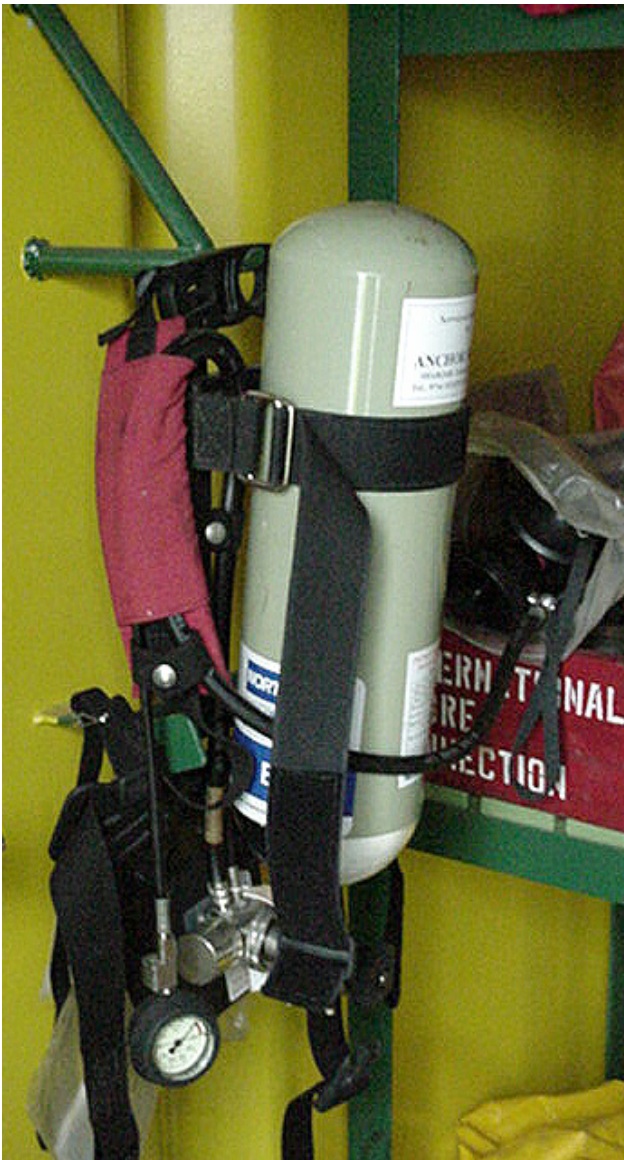
Good SCBA on brackets
