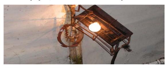
Particular care should be taken to provide suitable lighting for all access ways, deck openings, gangways and emergency escapes. If temporary lighting is in use it should be thoroughly checked and rigged in a safe manner, all cables should be secured to prevent further risk.
