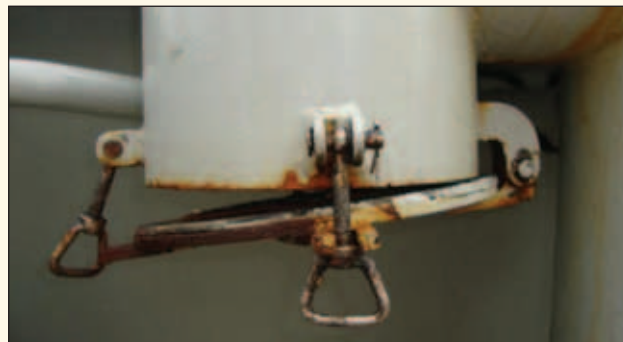
▲ Figure 3: Gooseneck vent with offset flap hinge
