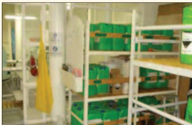
▲ Figure 7: Example of a well-laid out chemical storage area on board ship, showing PPE, placards and safety data sheets. Besides providing portable eye wash kits, it may be prudent to also provide an emergency shower and eye wash basin in the vicinity that can be operated by a temporarily blinded person: Editor
