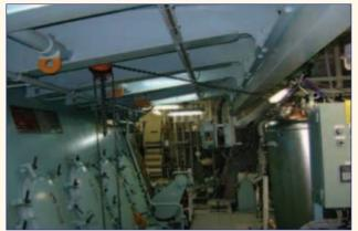
▲ Figure 2: View of unsafe arrangement of chain block showing hook chain leading sideways to OWS
