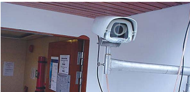
Here, it is possible to photograph all visitors to the vessel. Records are stowed on a disc or tape, and would be very useful during times of a security alert.
