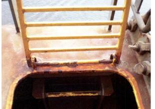
If visual inspection of these features reveals corrosion or wear, effective maintenance should take place at the first opportunity. It should also be noted that the wear to the protective paint coatings should be rectified quickly as these will precipitate the metal corrosion process if left untreated.
