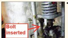
QCV disabled by inserting a bolt (Note: The bolt is partly painted, indicating it has possibly been there for some time.)
