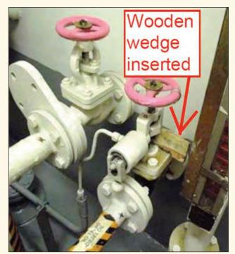
▲ QCV disabled by inserting a wooden wedge
