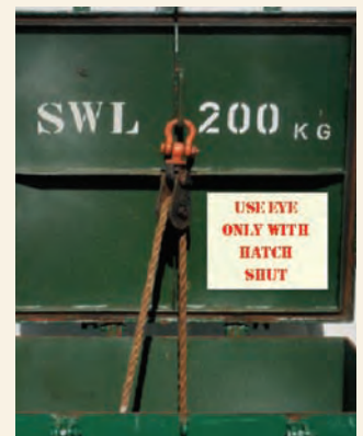
Dedicated padeye on underside of hatch lid intended for use only when lid is secured in closed position
