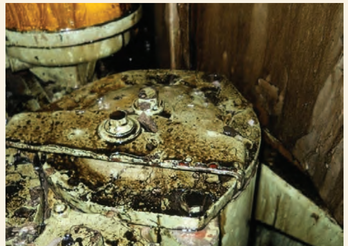
View of displaced fuel filter cover
