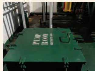
View of pump room hatch in shut position
