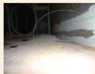
Buckled stringer inside side ballast tank caused by contact in bow region
